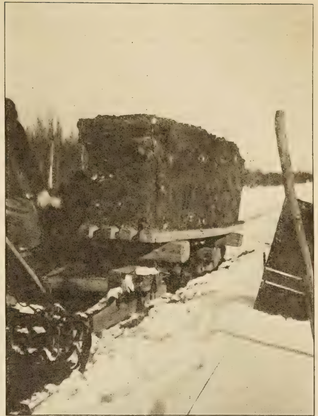
UNLOADING 7-YARD SLEIGH LOAD OF GRAVEL, FEDERAL-AID PROJECT 85, OCONTO COUNTY, WIS.
